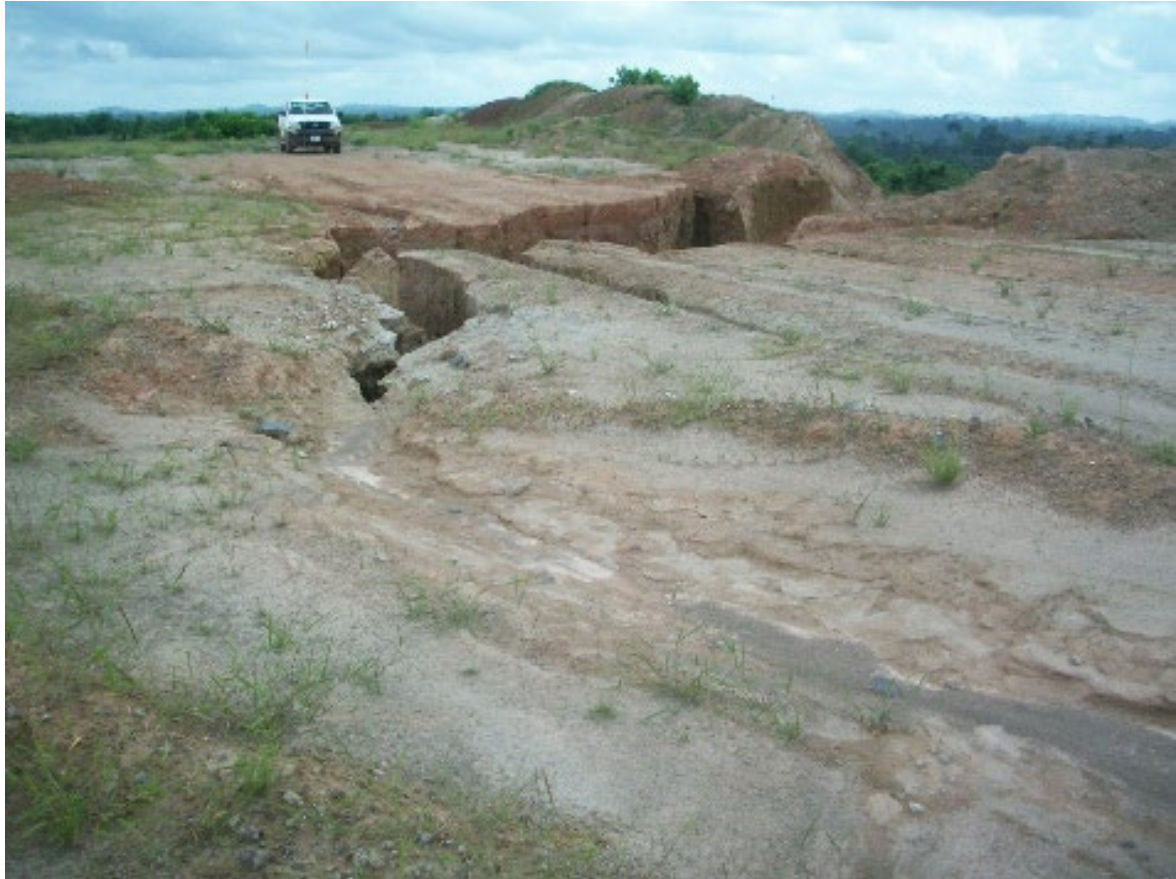
Figure 2: Failing embankments and sediment transports into tailings due to intensified rainfall
