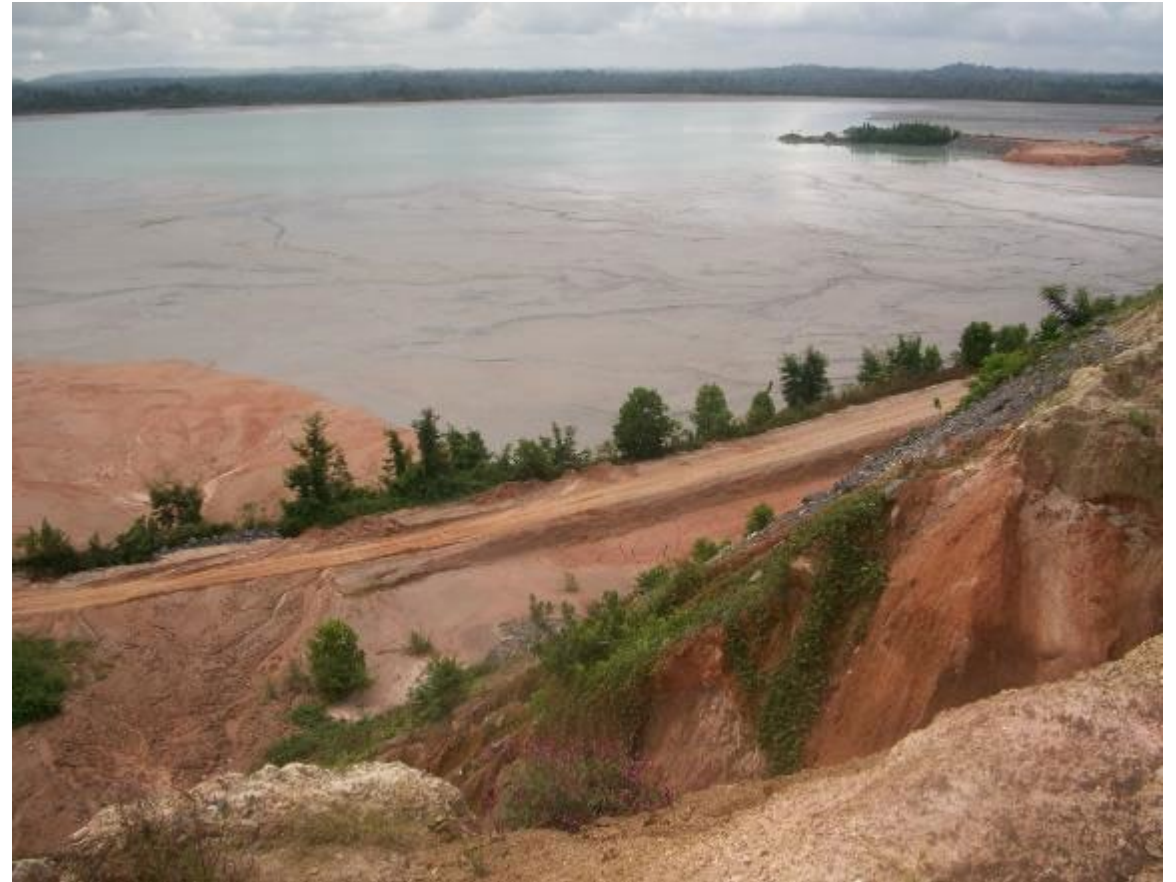
Figure 2: Failing embankments and sediment transports into tailings due to intensified rainfall
