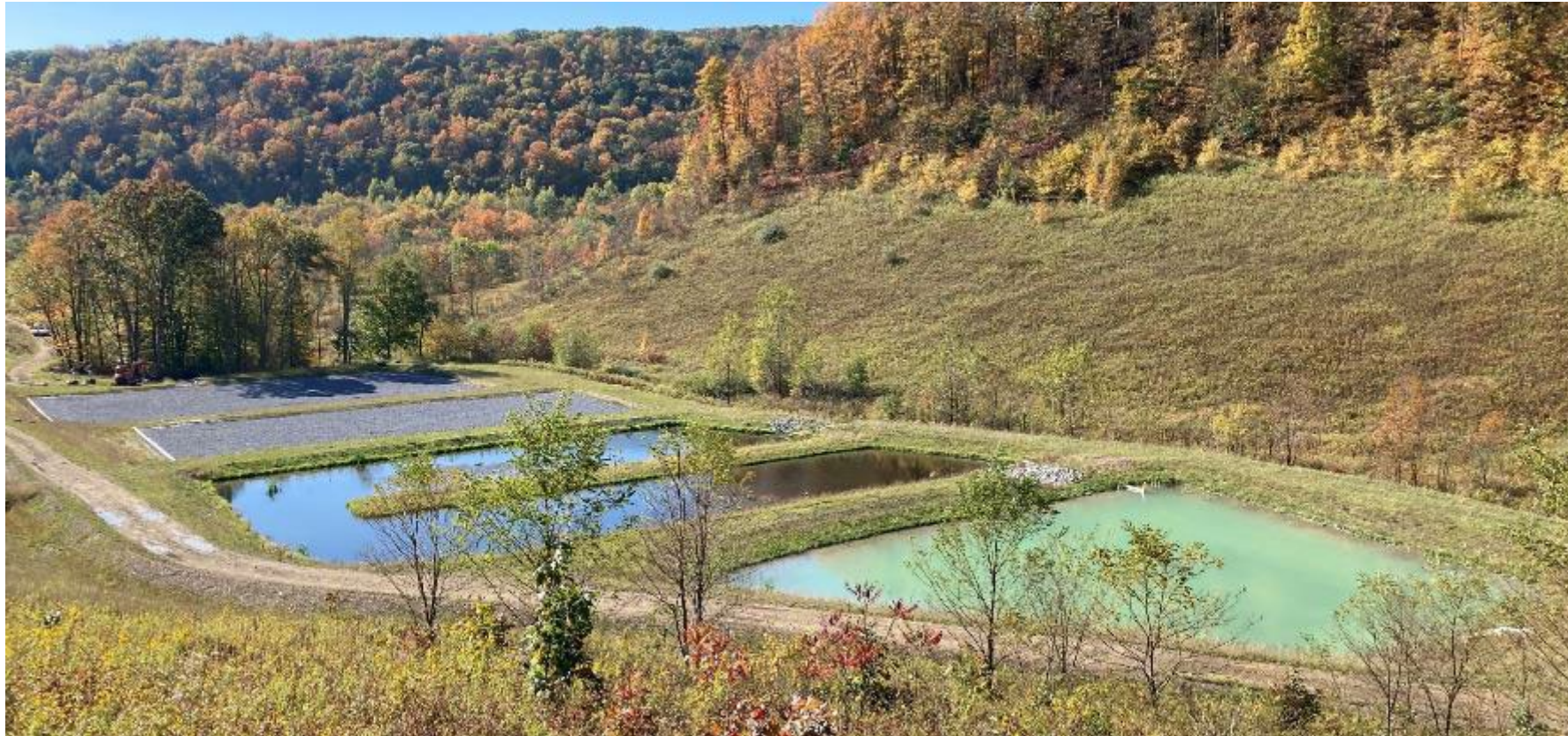
Cherry Run passive mine water treatment system (Elk County, PA)
