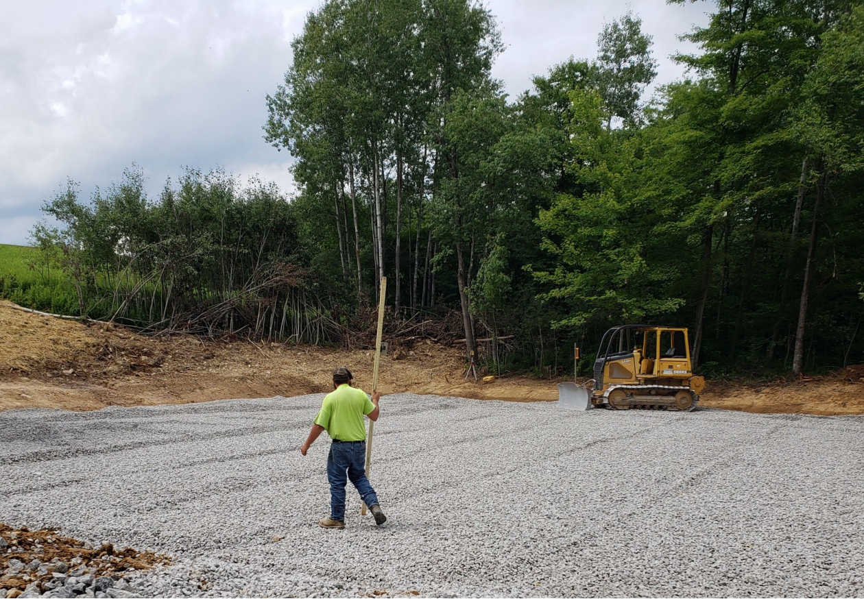
Limestone aggregate neutralizes acidity
