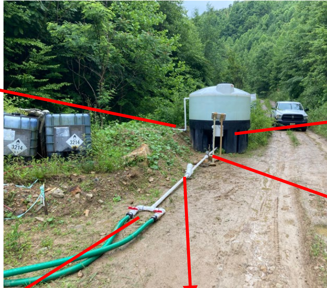
Tank 2 to geotubes
