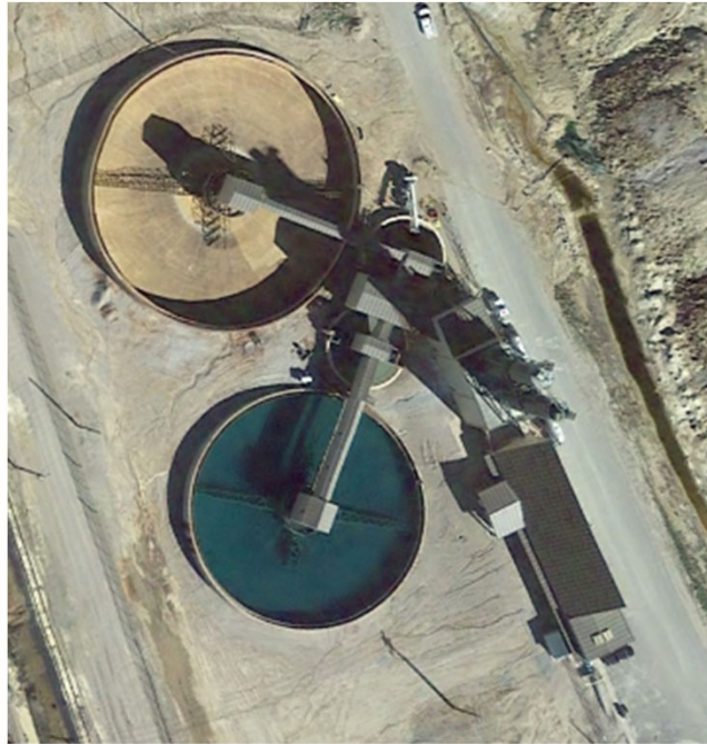
Horseshoe Bend AMD Plant
