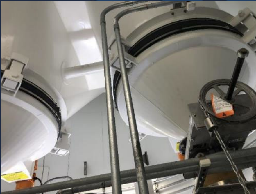
Inside the Lime Silo
