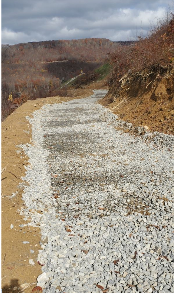
Construction and Operation of Iron Staining Bed
