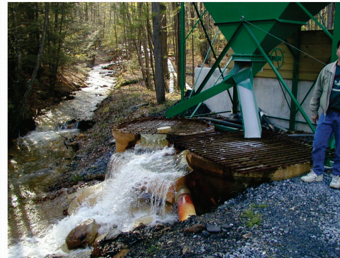
Limestone Diversion Wells
