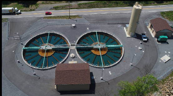
T & T AMD Treatment Plant
