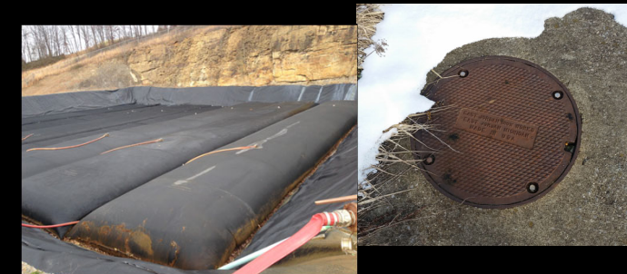
(6) Geotube Deep Mine Sludge Storage
