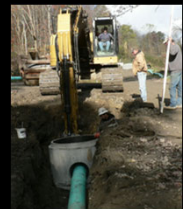
2.5 Miles of Pipeline
