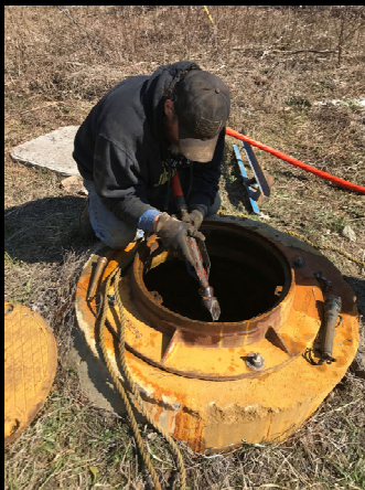
Cleaned by Regular Scheduled High-Pressure Jetting
