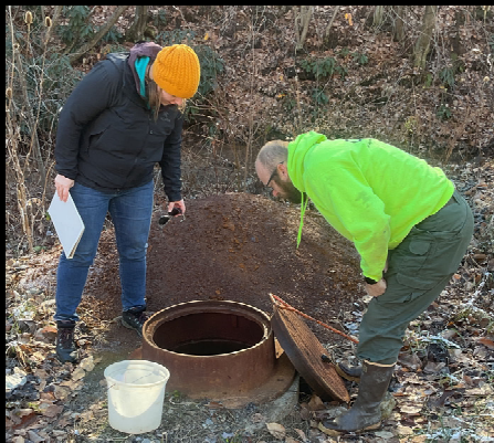
Grit Accumulation from Jetting & Settling
