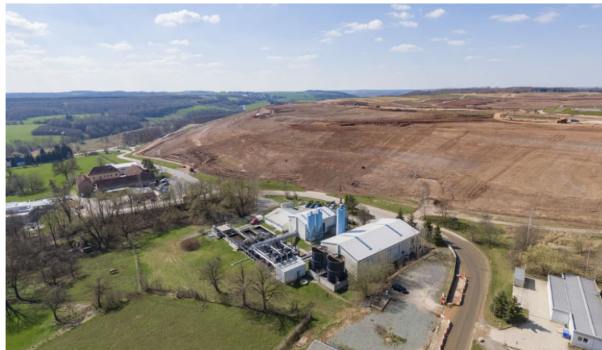
Tailing pond Culmitzsch and WTP Seelingstädt
