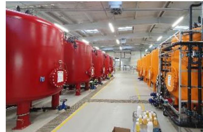
WTP Helmsdorf new: ion exchange / adsorption
