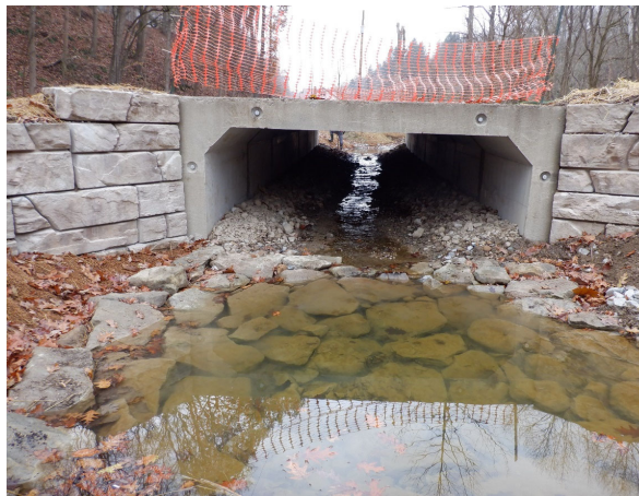
Outlet: As-Built Condition
