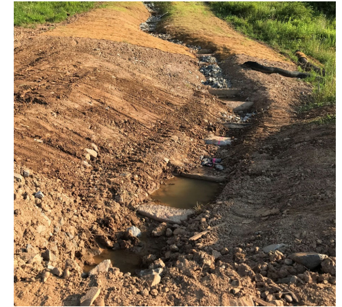
Step Pool Construction
