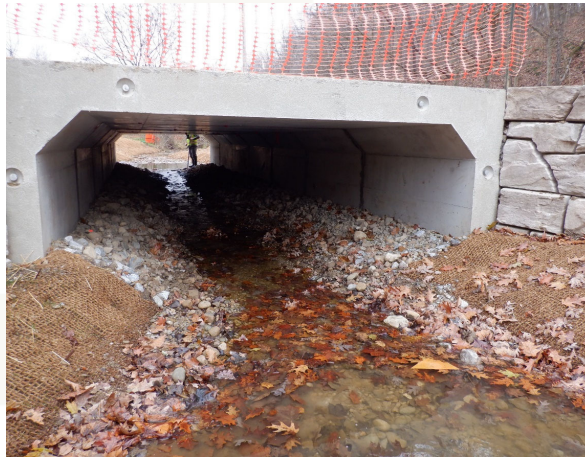
Inlet: As-Built Condition
