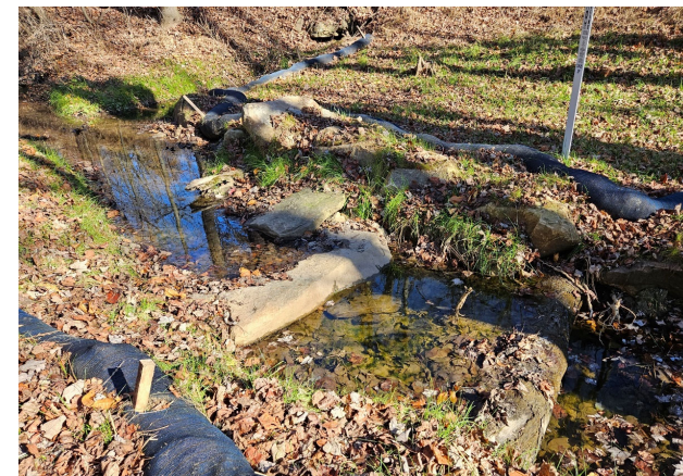
Constructed Restoration Reach
