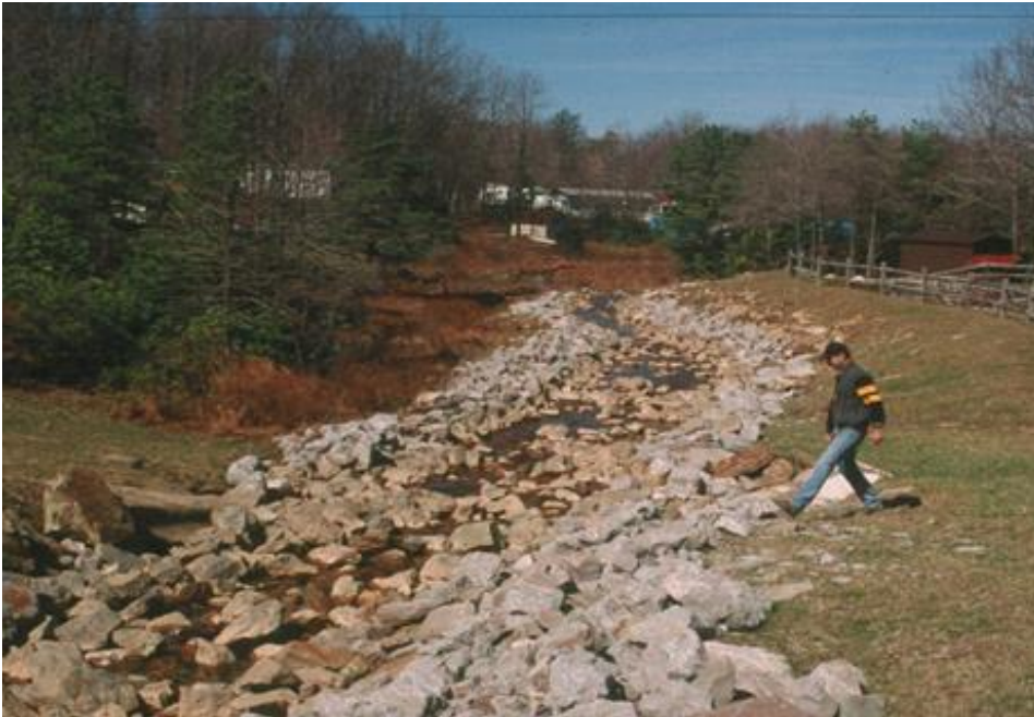
Figure 4. An open limestone channel (1995)
