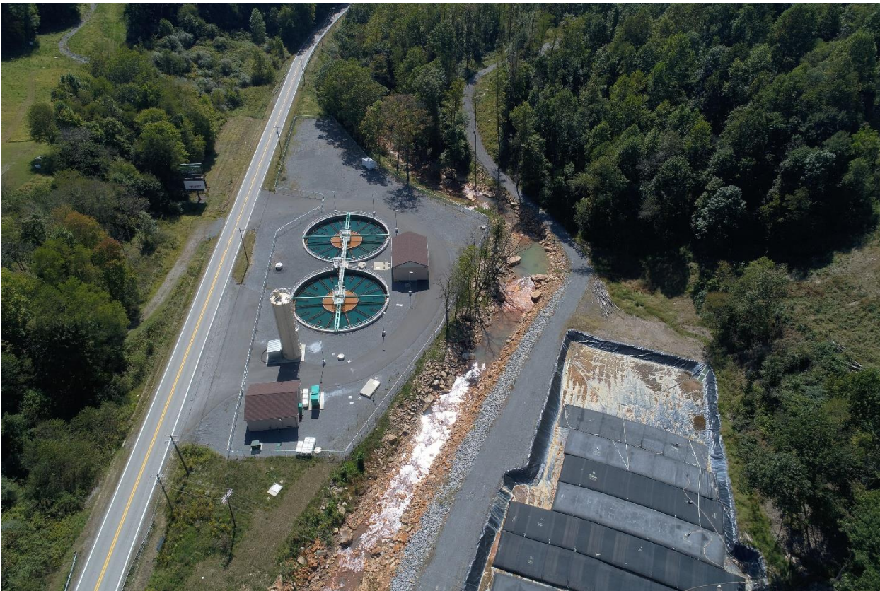
Figure 2. The West Virginia Department of Environmental Protection’s Muddy Creek AMD treatment plant near Albright, WV, showing the lime silo and system control building in the lower left, two clarifiers and Geotubes across the creek for collection and dewatering of AMD precipitates.
