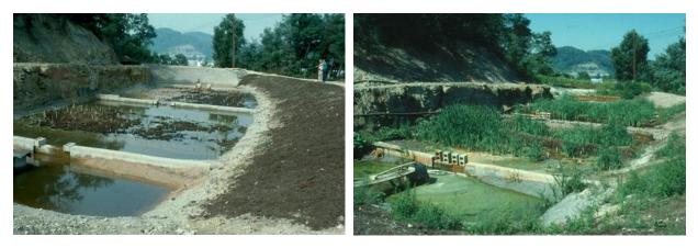
Figure 3A. A Typha-based wetland immediately after construction in West Virginia. B. the same site, two months later.
