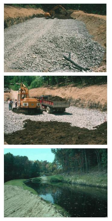
Figure 6. Construction of an early SAPS in 1995, which has subsequently also been referred to as RAPS, vertical flow ponds, and vertical flow systems. A. Initial placement of the limestone base layer with underdrain piping. B. Compost layer being placed on top of the limestone. C. The system filled with water.
