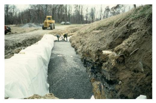
Figure 5. An anoxic limestone channel being constructed, soon to be covered with plastic sheeting and a soil cover.
