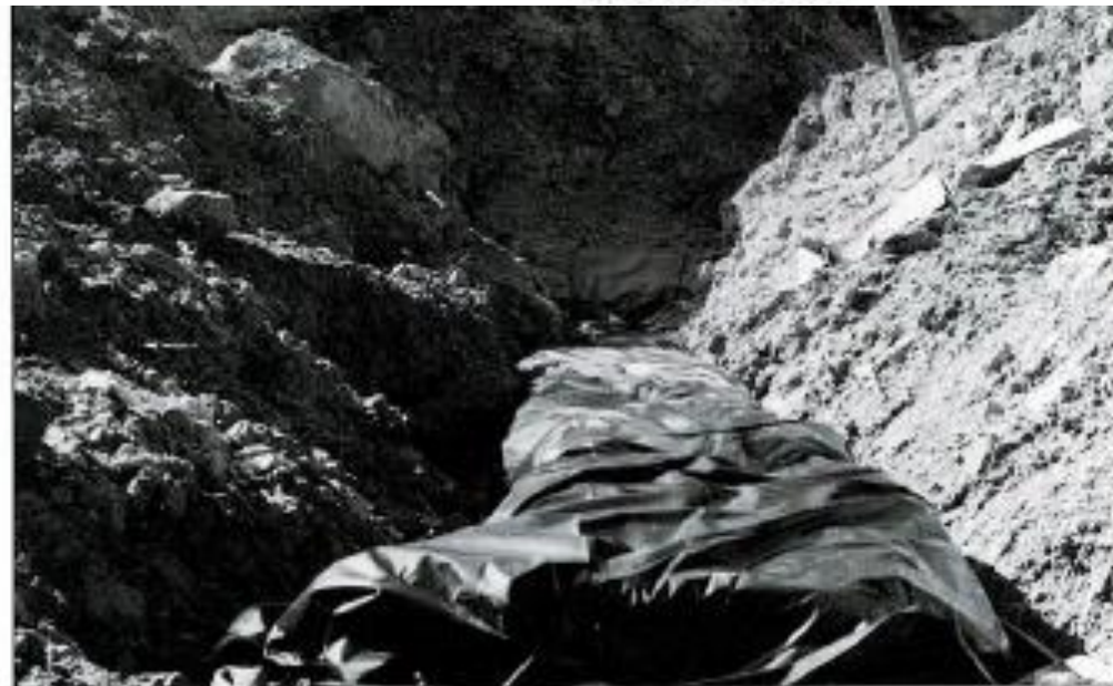
Figure 3. The limestone and hay in the trench were covered with plastic.
