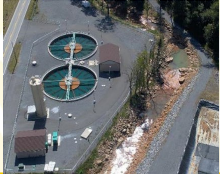
Muddy Ck AMD plant
