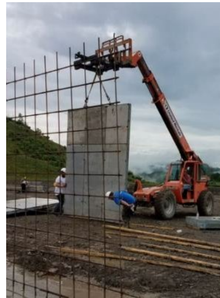
Marion Branch Industrial Park Worksite in Kentucky
