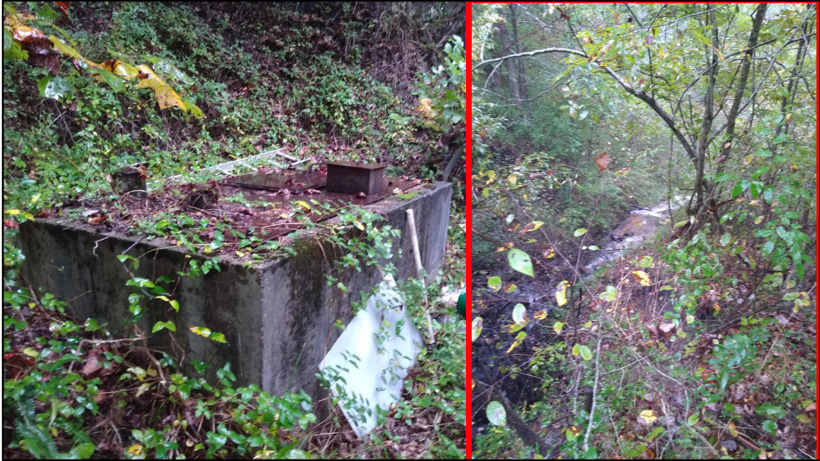
The mine portal is secure with a splitter box that allows for overflow to the creek. It was developed by Edsell Reddin in the late 1980's.
