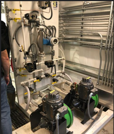
(1) Lime Slurry Injection for pH Adjustment
