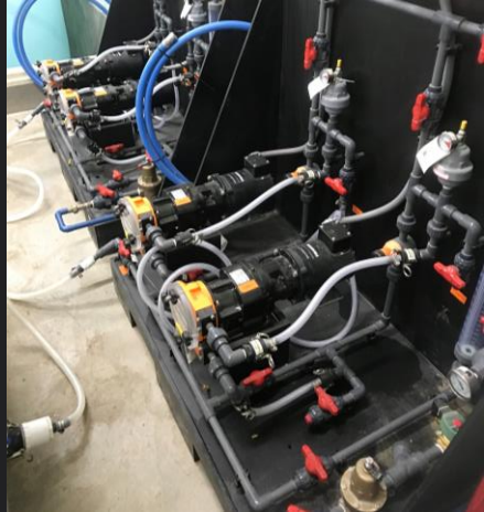
(2) Polymer Injection Aid Flocculation
