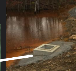
AMD AML Lagoon Drop Inlet
