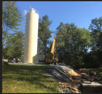
Glade Run In Stream Dosing Unit
