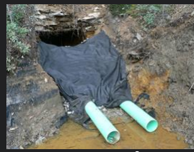
Listen AML Deep Mine Wet Seal
