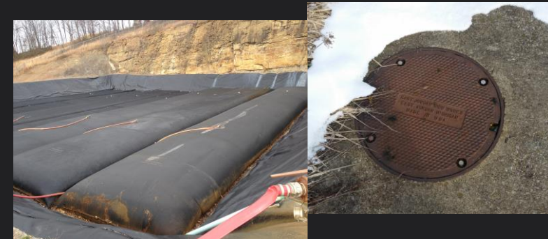
(6) Geotube Deep Mine Sludge Storage
