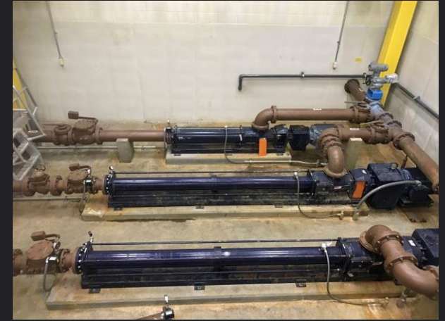
(5) Sludge Pumps to Mine or Geotubes
