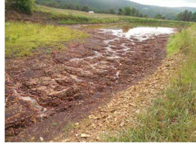
Figure 2. Typical AMD treatment pond where precipitates are captured and allowed to settle from treated AMD.
