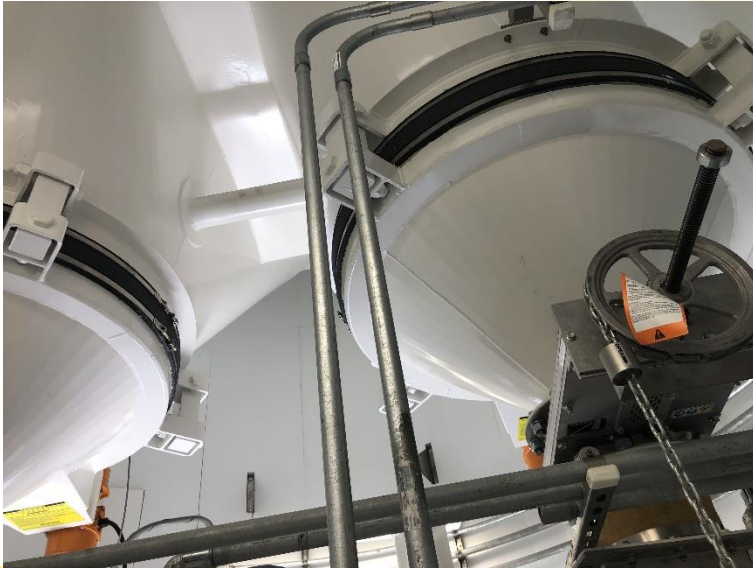
Inside the Lime Silo
