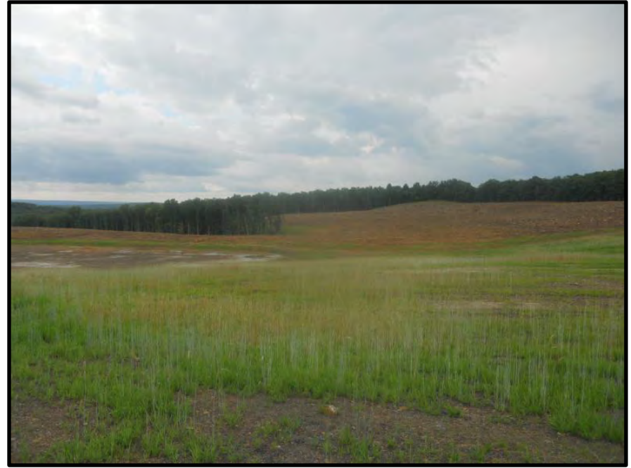
Figure 32 – (June) Post-Construction, Conventional Backfill Area and Pond
