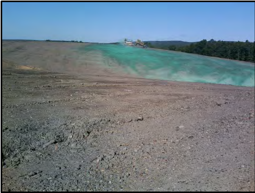
Figure 30 – During Construction, Seeding of Conventional Backfill Area
