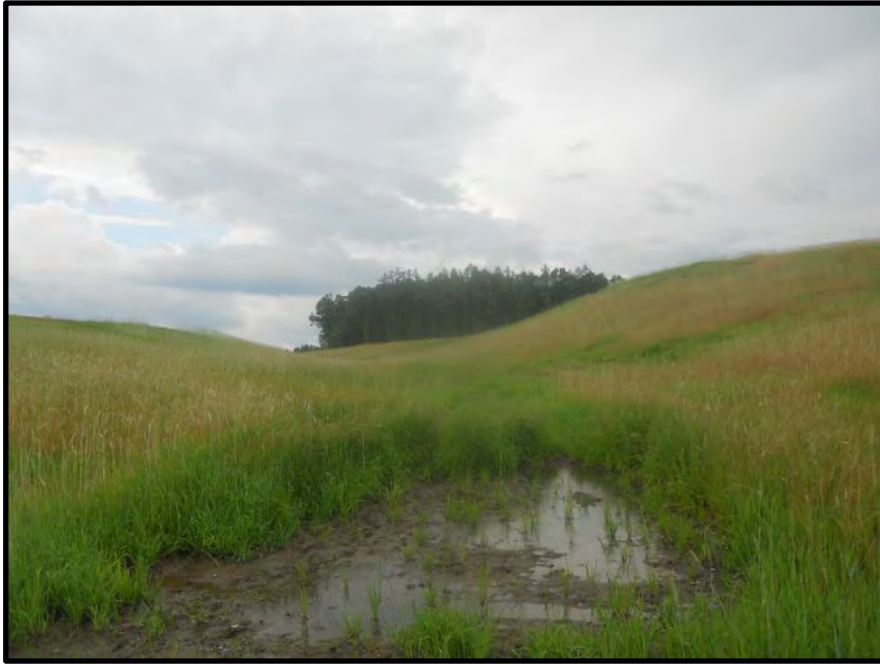
Figure 34 – (June) Post-Construction, Conventional Backfill Area
