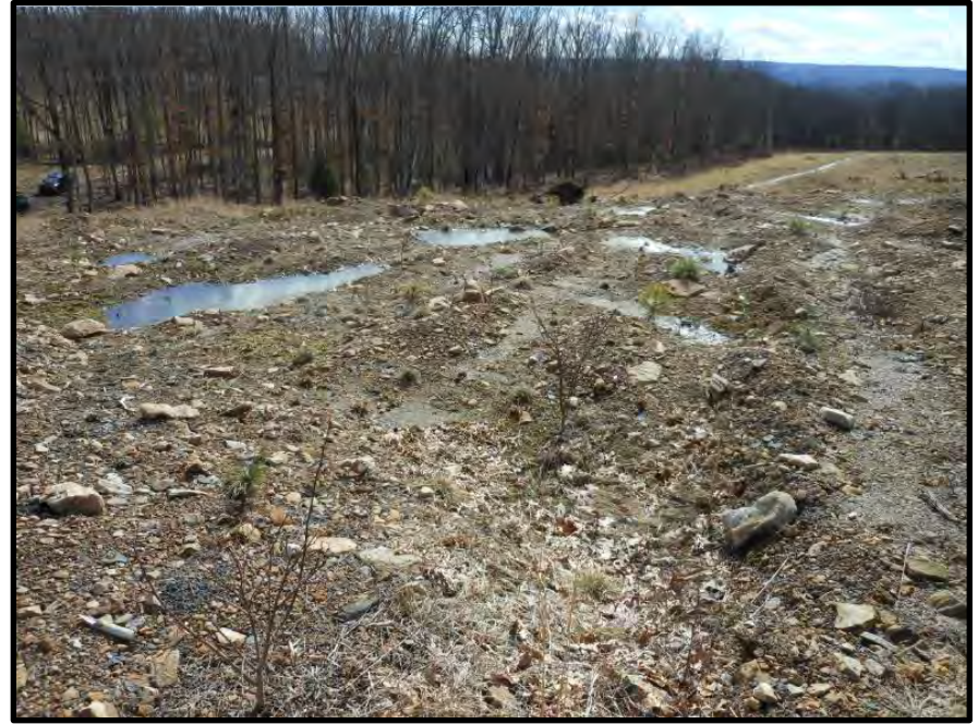
Figure 36 – (March) Post-Construction, FRA Grading and Tree Seedlings
