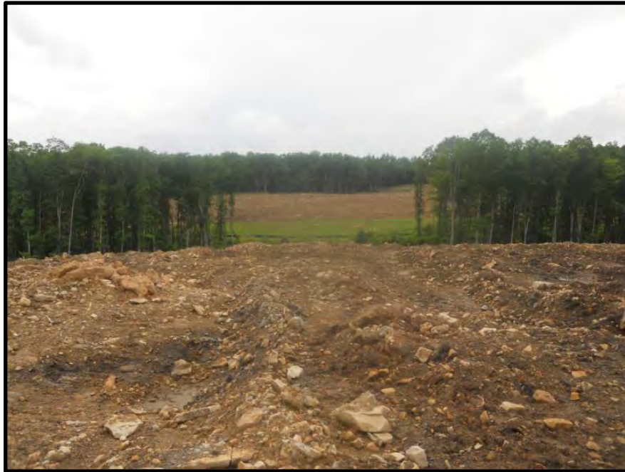
Figure 31 – During Construction, FRA Grading Prior to Tree Seedlings Planting
