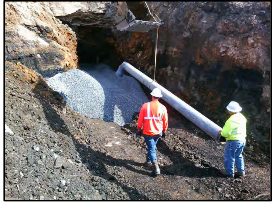
Figure 25 – During Construction, Deep Mine Wet Seal and Subsurface Drain
