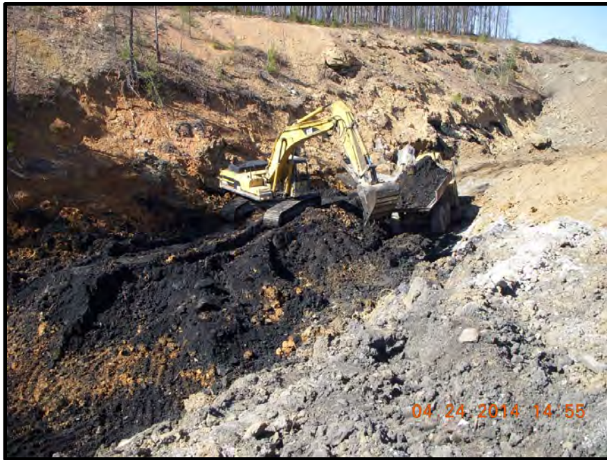
Figure 23 – During Construction, Buried Coal Refuse Removal
