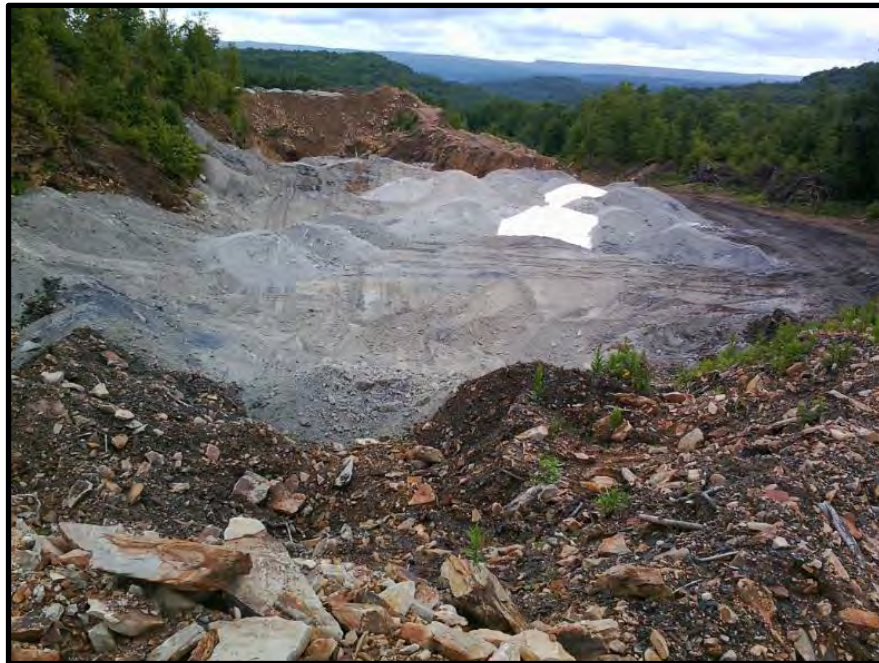
Figure 27 – During Construction, Alkaline Addition
