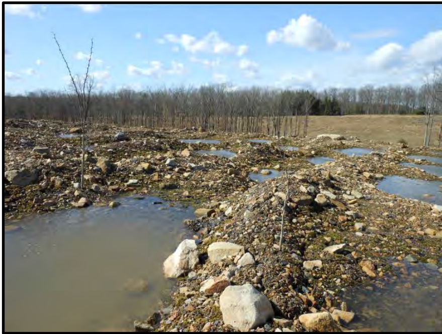
Figure 35 – (March) Post-Construction, FRA Grading and Tree Seedlings
