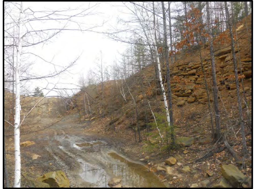
Figure 20 – Pre-Construction 2012 Typical Dangerous Highwall
