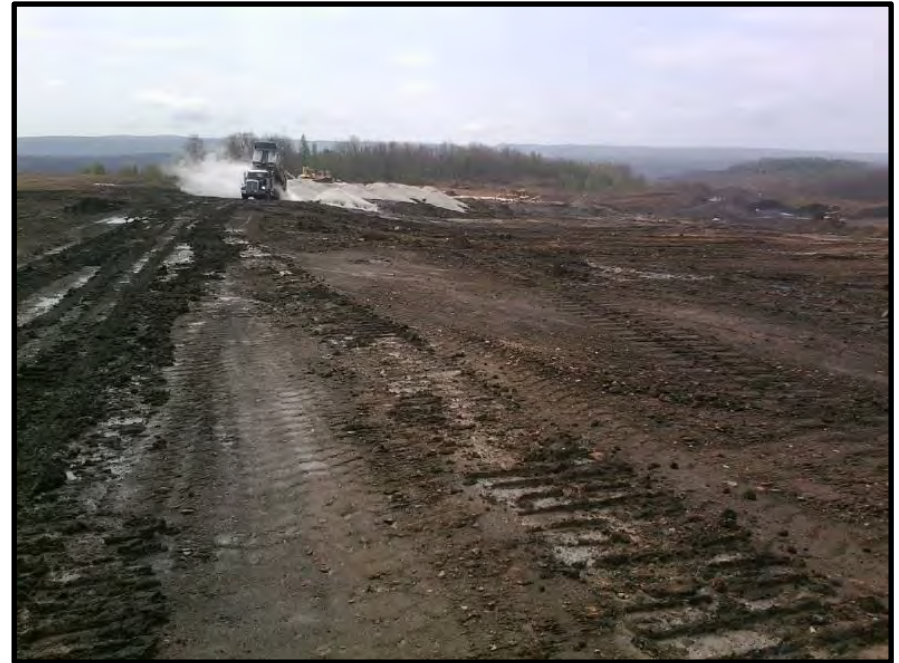
Figure 29 – During Construction, Backfilling and Alkaline Addition Blending
