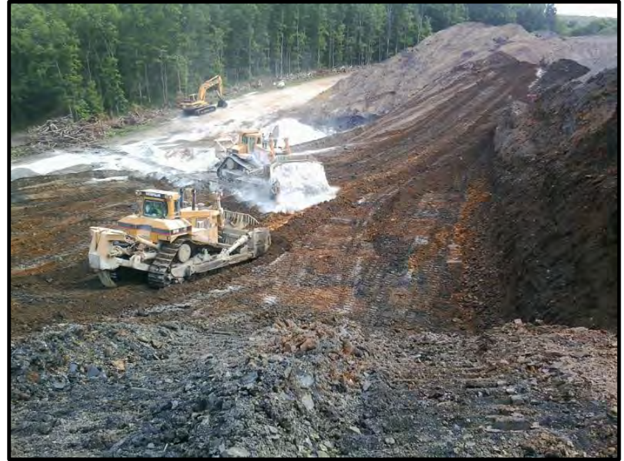
Figure 28 – During Construction, Backfilling and Alkaline Addition Blending
