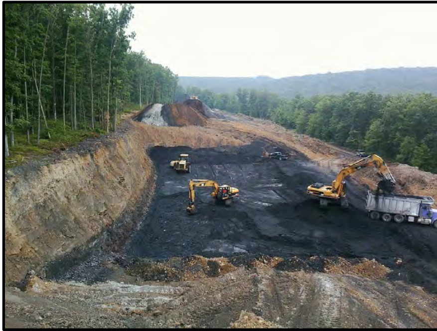
Figure 22 – During Construction, Coal Removal
