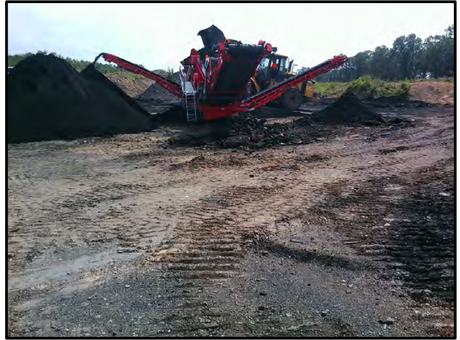
Figure 24 – During Construction, Coal Screening
