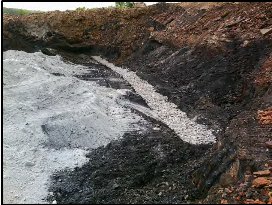
Figure 26 – During Construction, Rock Underdrain
