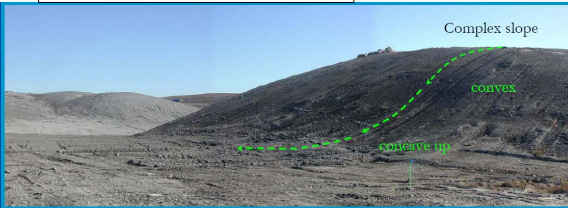
Graded slope at North Antelope Rochelle Mine (Anna Waitkus, 200)
