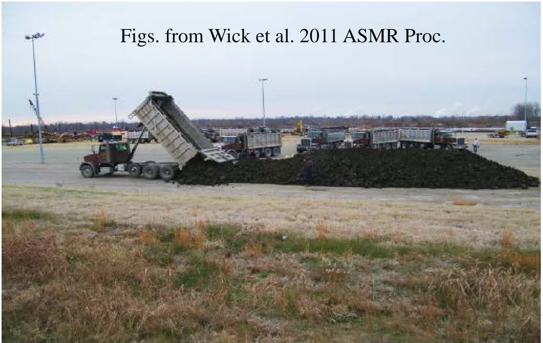
Figure 1. Maryland Port Administration Cox Creek Facility dredge material being placed at Port Tobacco, Shirley Plantation, Charles City, VA, in November of 2009. The materials were immediately covered with a tarp to limit rainfall additions and oxidation.
