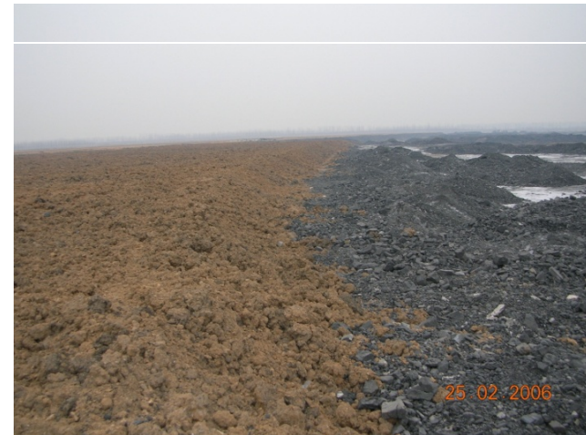
Filling reclamation with coal wastes
