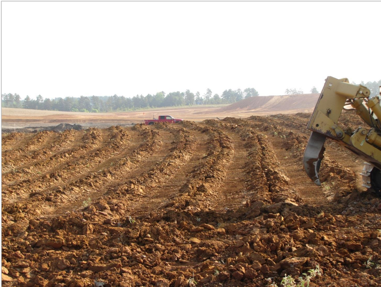
Single vs Cross-Ripping (90 cm depth)
