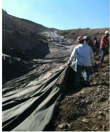
Placement of the fabric wrap for the under drain was labor intensive and time consuming.
