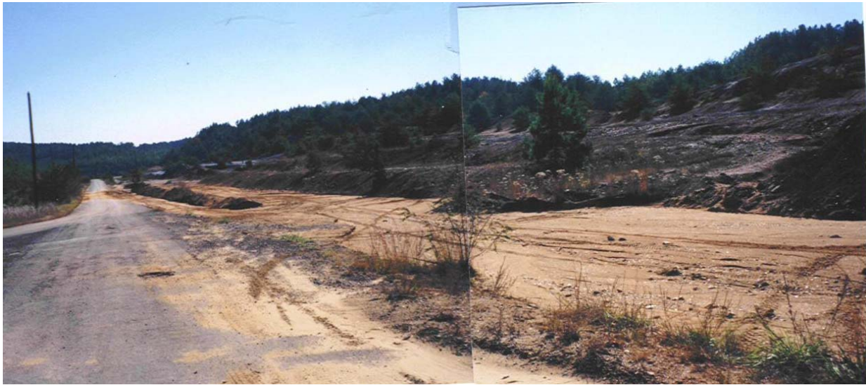
Figure 3. Silt from eroded areas at wetland construction site (well above flood plain).
