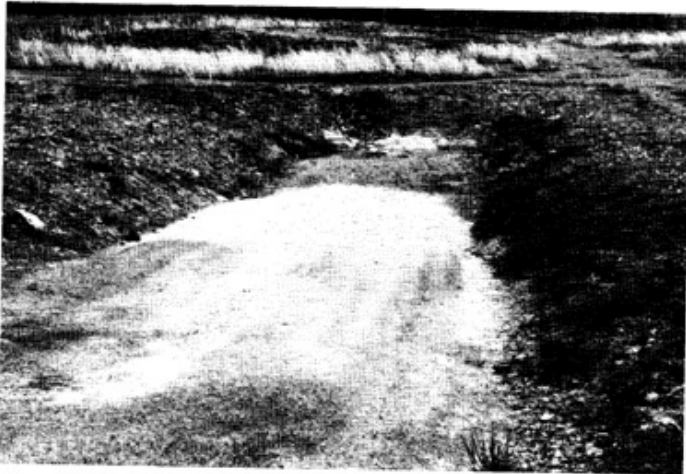
Figure 8: The alkaline trench concept advocates surface water infiltration into the backfill. This trench is packed with sodium carbonate briquettes and limestone chips which will cause the water to be highly alkaline as it enters the backfill.
